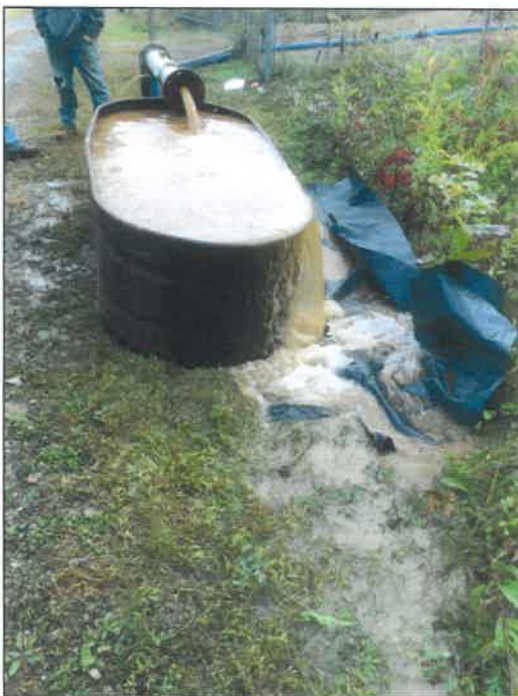
Iron, manganese, and sediment removal by pumping and surging (left – 10/4/2019) and decrease in sediment and iron/manganese (right – 10/8/2019)
