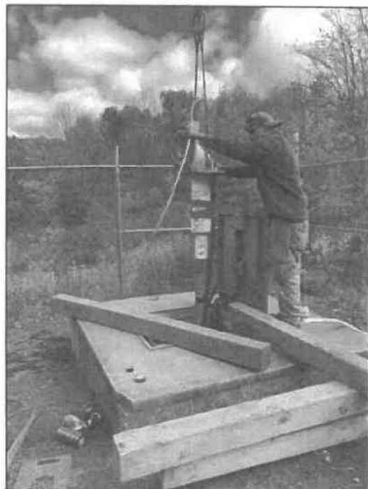
Reinstallation of pump and motor (left) and column piping and stilling wells (right) - 10/18/2019
