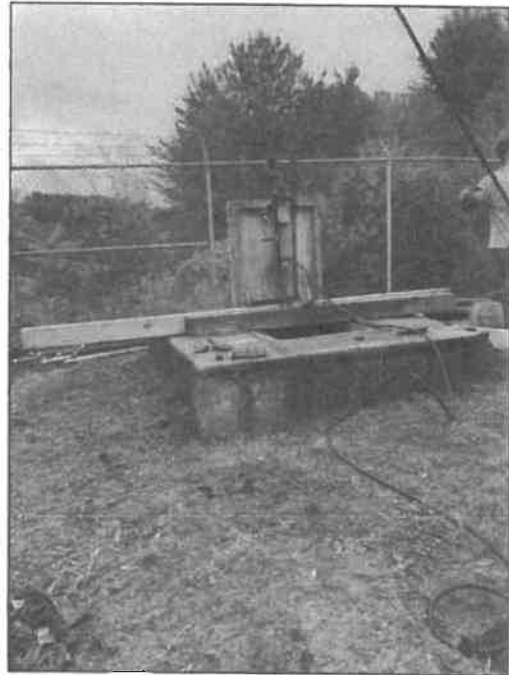
Installation of inflatable packer and AquaFreed injection equipment - 10/1/2019
