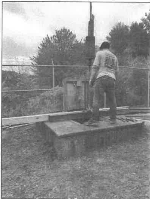
Installation of inflatable packer and AquaFreed injection equipment - 10/1/2019
