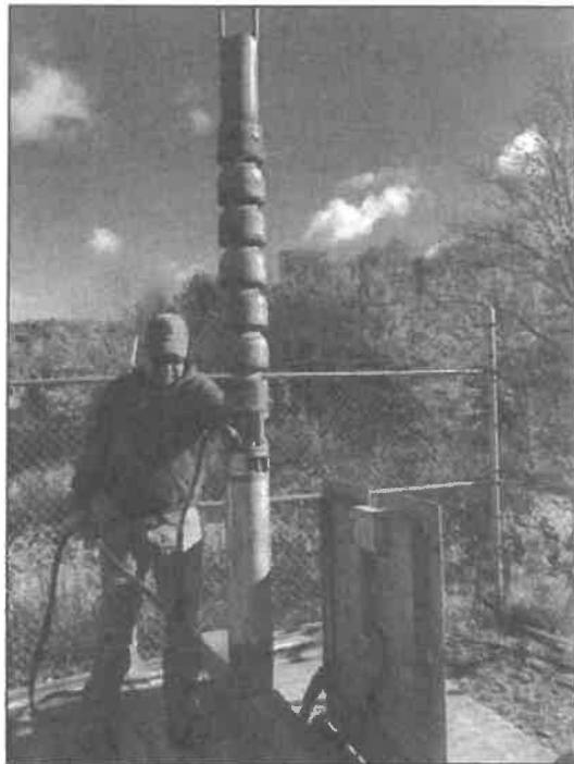
Reinstallation of pump and motor (left) and column piping and stilling wells (right) - 10/18/2019
