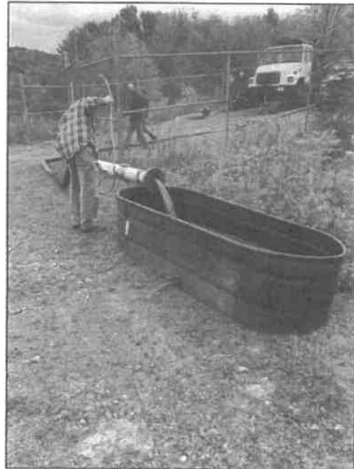
Installation of surge blocks and equipment (left) and initial surge of Bedrock Well #2 (right) - 10/1/2019
