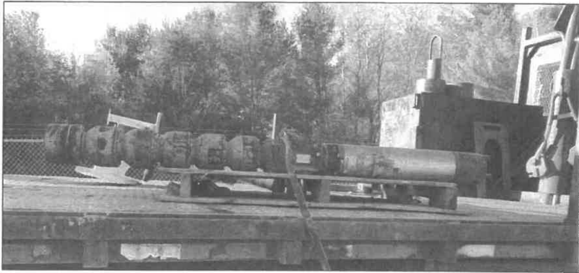
Steam cleaned and inspected pump and motor returned to Bedrock Well #2 - 10/18/2019
