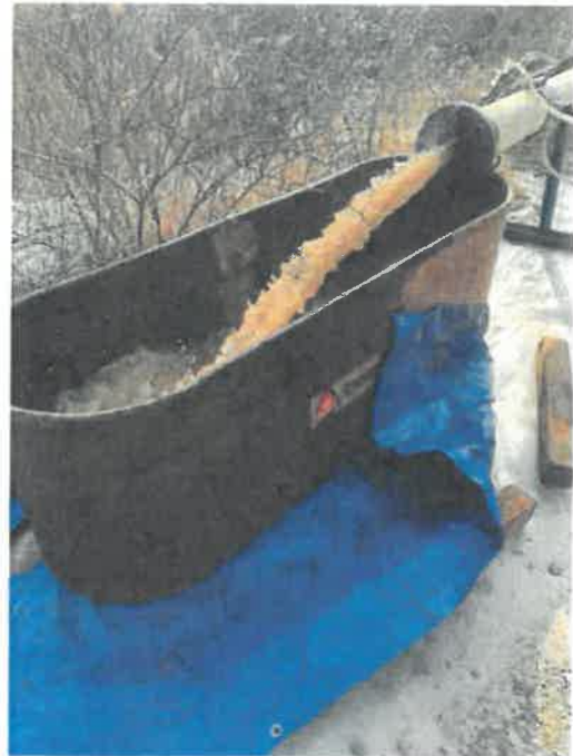
Iron, manganese, and sediment removal by pumping and surging (left – 1/21/2022) and decrease in sediment and iron/manganese (right – 1/25/2022)
