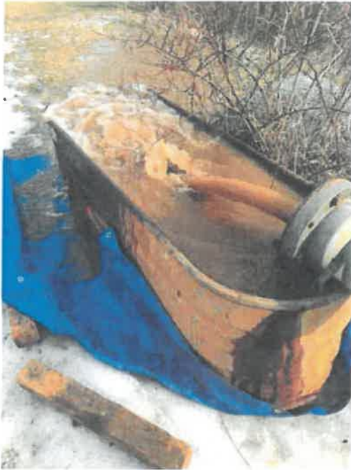
Iron, manganese, and sediment removal by pumping and surging (left – 1/21/2022) and decrease in sediment and iron/manganese (right – 1/25/2022)
