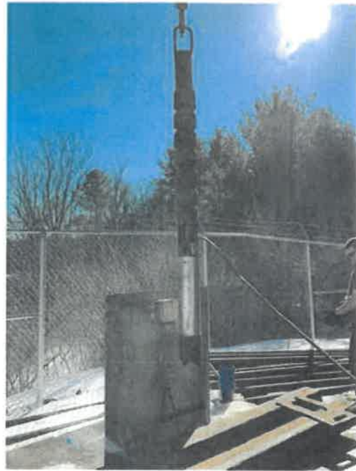
Steam cleaned and inspected pump and motor returned to Bedrock Well #2 -12/9/2022
