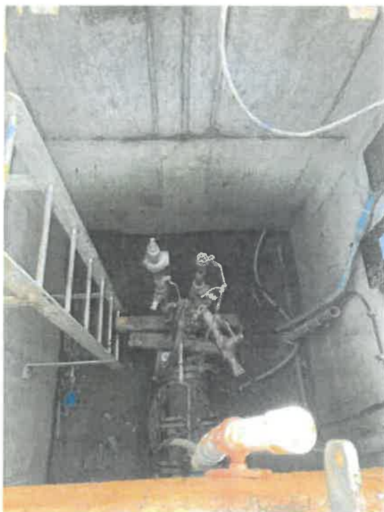
Christensen 6CLC-5 Pump and Centripro 15 HP Motor (left) and clogged intake screen - 1/12/2022
