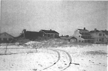
Photo 3: Vicinity of Suncook/Hooksett Streets, Looking Northwest
