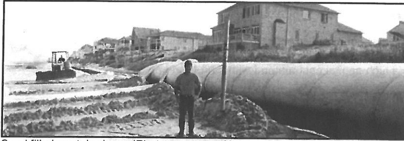
Sand filled geotube berm (Photo courtesy of Bradley Industrial Textiles, Inc.)
