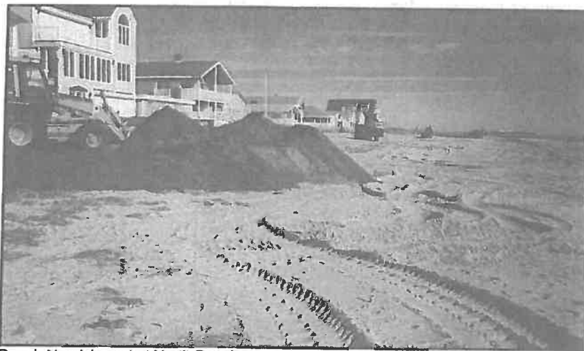
Beach Nourishment at North Beach
