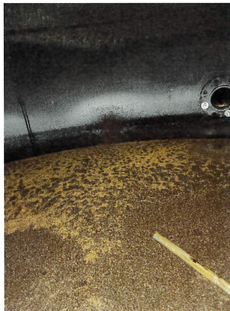
Figure 2 - Example of media surface in filter 3 (2230). Flat and generally free of debris
