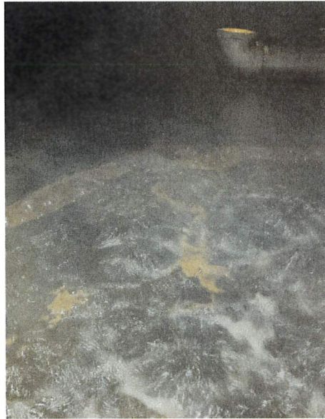
Figure 2: Air Scour pattern from filter #3 (2230)
